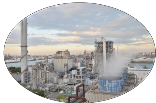
Gas turbine (thermal power plant)
